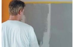
**Step 2**Apply the paint with a fleece roller to get a good layer thickness. Spread the paint well to ensure an even magnetic attraction force. Apply two or more coats.
