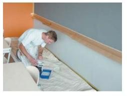
**Step 4**After 24 hours you can paint over the magnetic paint with a water-based paint in any colour.
