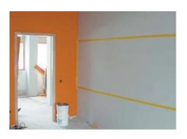
The more coats you apply, the stronger the magnets will adhere. Test the magnetic force of the wall after the second coat and if necessary apply a third coat. Do not sand down the painted surface: the iron particles will come to the surface and no longer be protected by the paint.
